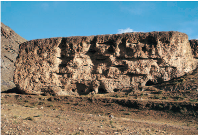
Fig. 4 The rammed mound of Tibetan mausoleum No.19
