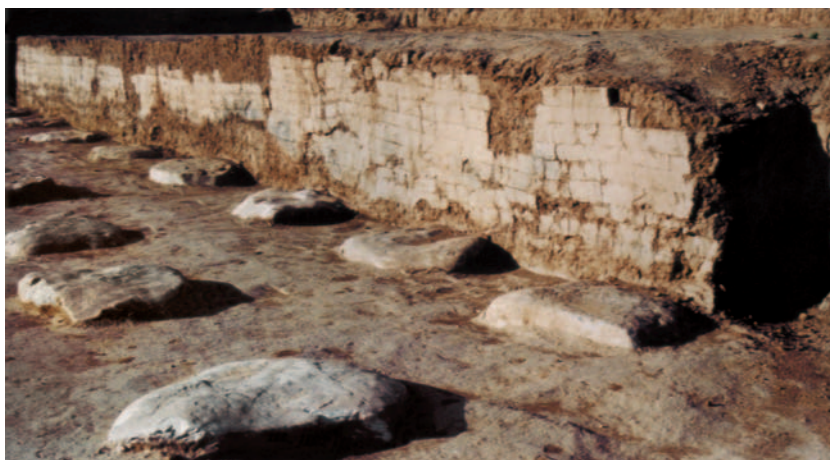
Fig. 4 Western rammed wall of the Western Han pier storehouse
