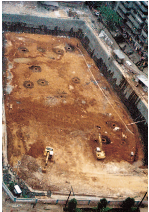
Figure 1. On-the-spot excavation of Dongpailou site
