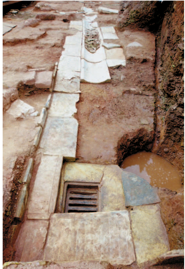
Figure 8. Open ditch and floor drain of the Nanyue Kingdom period (photo taken from south to north)
