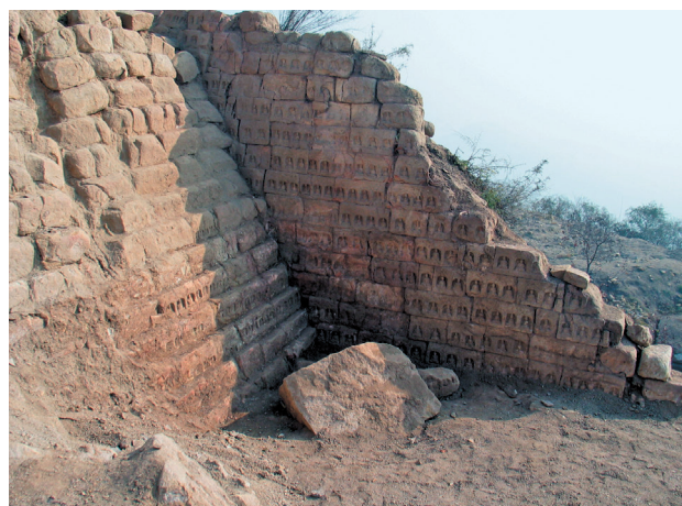
Figure 8 The eastern wall and the north section of the retaining wall seen from the inner side of the Giant Buddha Pavilion (W–E).
