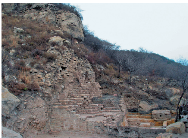
Figure 7 The eastern wall of the earlier phase and the retaining wall of the later phase of the north part of the porch of the Giant Buddha Pavilion (S–N).
