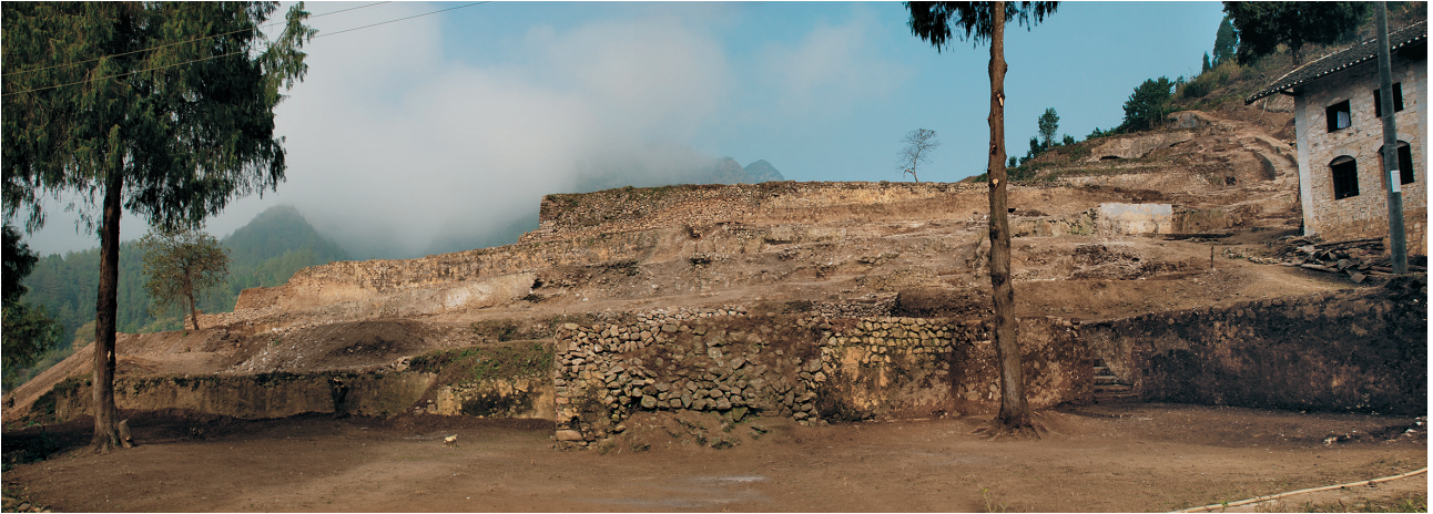
Figure 2 Southern wall of the palace area (S-N).
