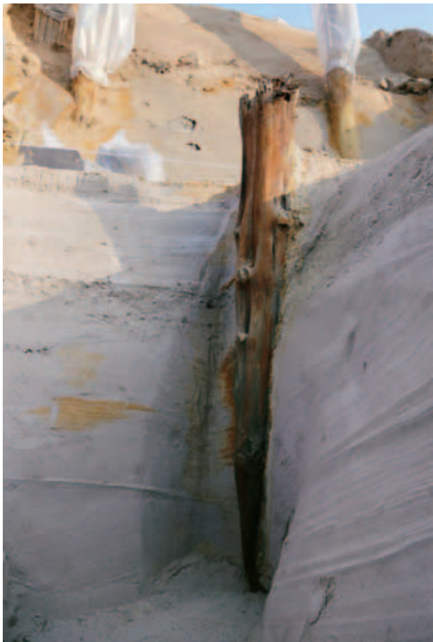
Figure 5 The piles of the Chucheng Gate Bridge No. 1 driven into the riverbed (W-E).
