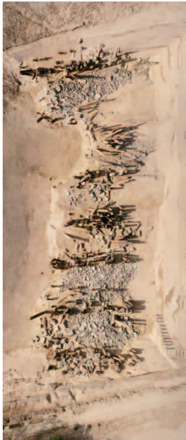
Figure 4 The orthophoto of the Chucheng Gate Bridge No. 1 (top is north).
