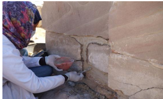
Fig. 13 During filling the joints and the gaps with new lime mortar © MTP
