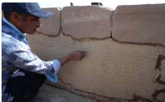
Fig. 13 During filling the joints and the gaps with new lime mortar © MTP
