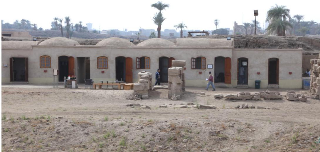
Fig. 15 New offices and storerooms on the site © MTP
