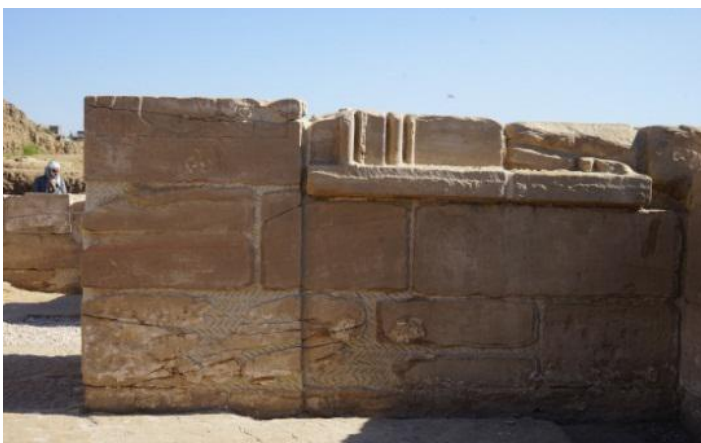
Fig. 14 Photos explains walls condition before and during restoration processes © MTP
