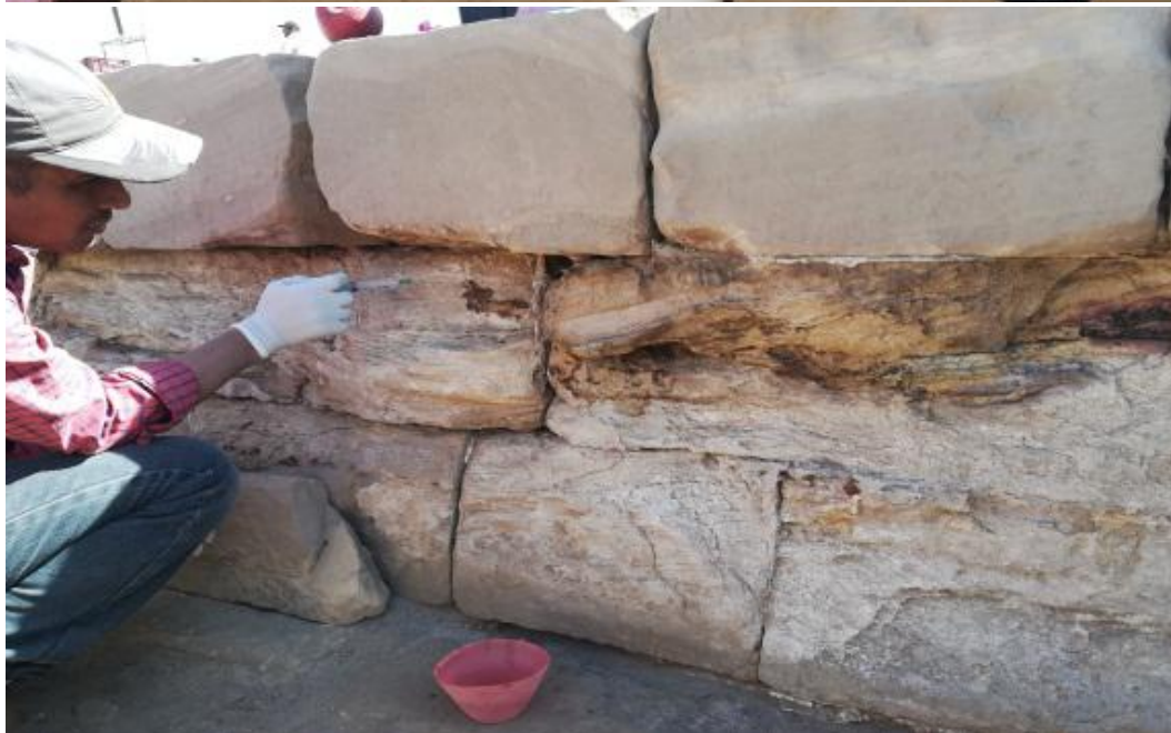
Fig. 11 During apply consolidation process at CH2 sandstone blocks © MTP
